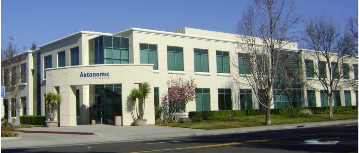
Typical two-story industrial/R&D warehouse style building.
