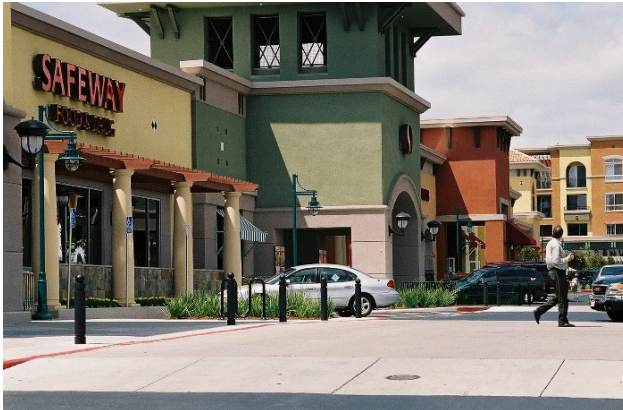
Retail center that provides pedestrian speed table in front.
