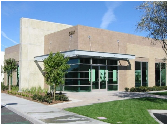
Utilitarian architecture is appropriate for industrial districts.
